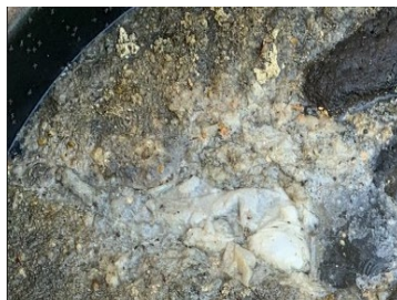
Wipes & Grease in a grinder pump
